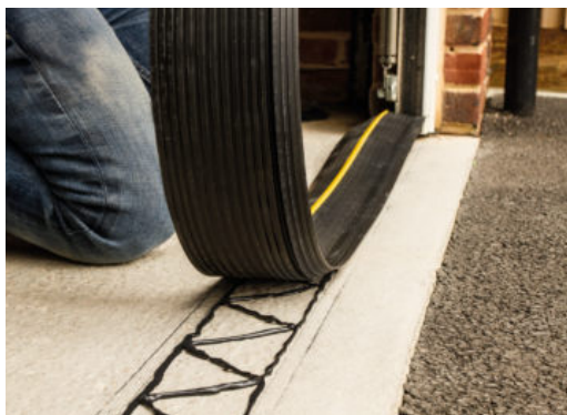
Installation of Weather Defender
