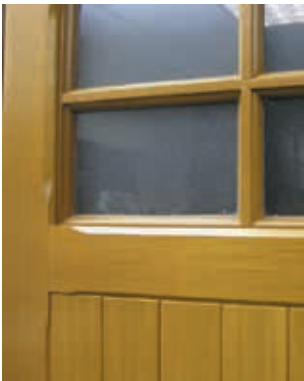
Glazing details of a Sherwood Southwell showing glazing bar details, the windows in this door are a solid window sash inserted into the door panel as shown
