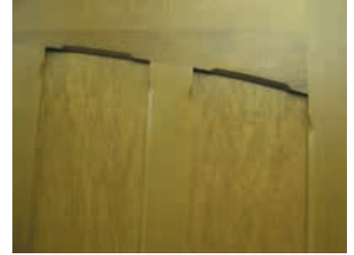
Panel detail of plywood panelled doors with cedar facings showing stopped chamfer profile
