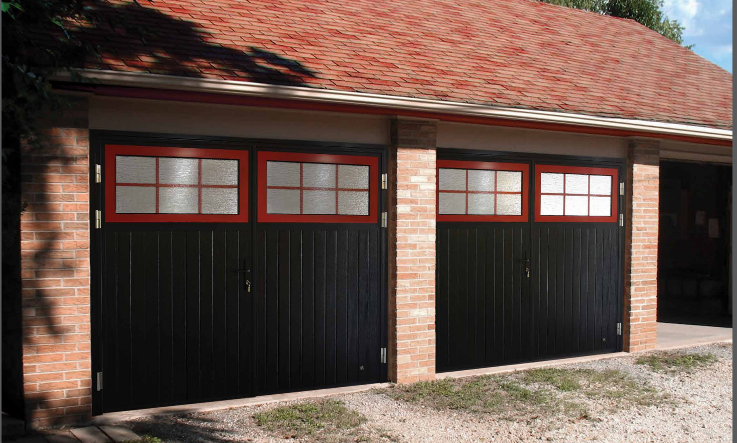
Glazing panels in contrasting 'Flame red' colour.
